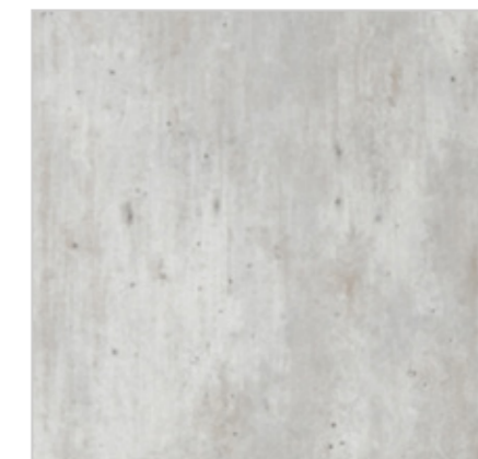
Cracked Cement Code: 2204-M00
